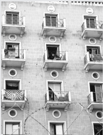
Case al check point
